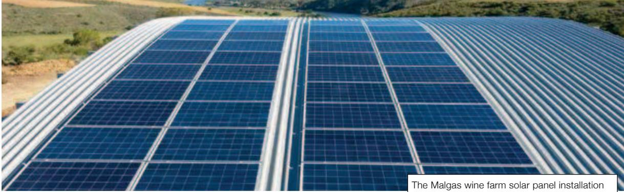
The Malgas wine farm solar panel installation on a metal roofing system.
