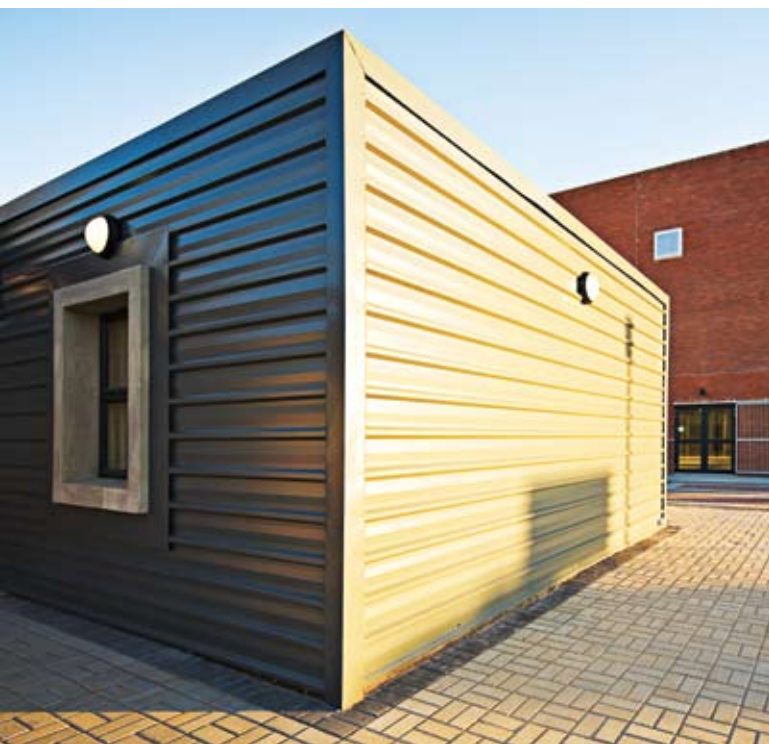
Main picture & below: Trimflute® used as roofing and cladding on the Govan Mbeki Sport Centre. project.
