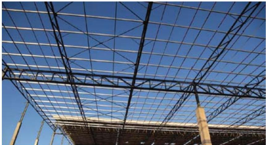
Above: Metsec purlins of 202 mm web depth x 1.6 mm thickness spanning 8.0 mtr. Test certificates are supplied for the high yield strength steel which is used in forming these ultra-light sections.
