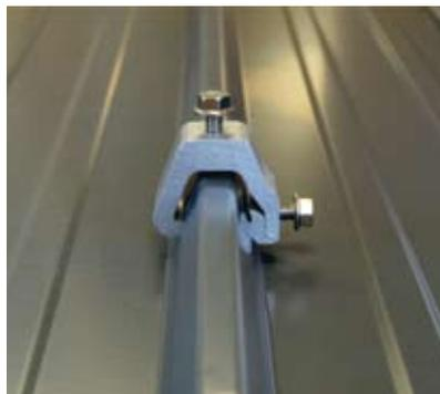
Left: Saflok 700 roof sheet with S-5 clamp – the use of S-5 clamps will not void the warranties on concealed fix sheeting because they are non-piercing. The patented clamp design has been tested to over 1,000 kg pull out value.
