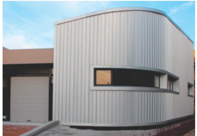
The male rib is to include spurs to ensure a double interlocking action with adjacent sheets. The minimum sheet depth shall be 41mm. Two stiffening ribs are incorporated in each pan.
